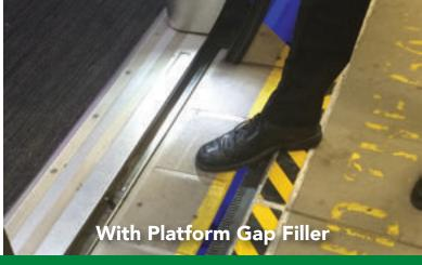
Platform Gap Filler is an engineered sturdy, hard-wearing rubber profile that is mounted along the edge of a train platform to reduce the gap between the platform and the entrance of a passenger train; ensuring that when a train has stopped at a platform, passengers are able to enter and exit with safety.
